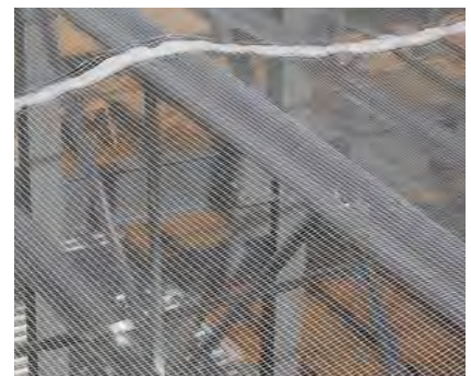
Sky-Web® and Sky-Web II® do not eliminate fall hazard from the non-leading-edge perimeter of the roof during installation.
